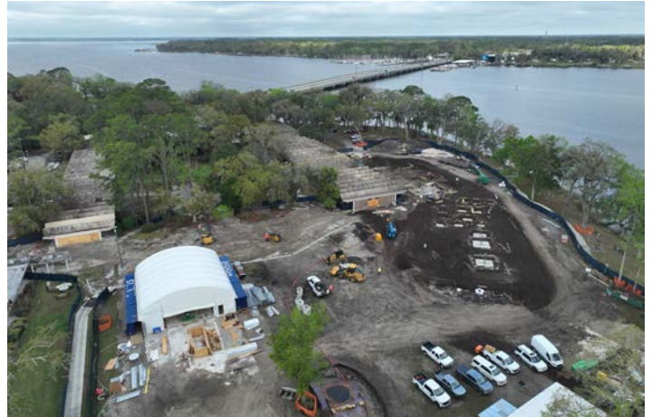
A birds-eye view of the progress being made on The Woodlands at Westminster Woods on Julington Creek.
